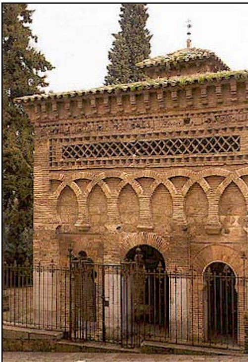
Figure 11: Façade of bab Mardum (999-1000) showing the Cordoban intersecting arches while the entrance is marked by the three famous Muslim arches, from left to right; The cinqfoil, the semi-circular, and the horseshoe.
