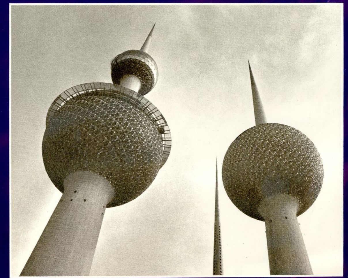
Water Towers Kuwait City, Kuwait
