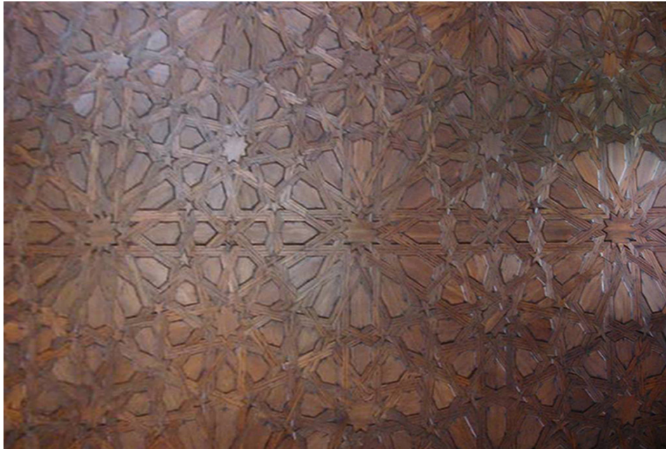
Figure 1. Wooden ceiling panel in El Mexuar
